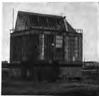
The Experimental Building
